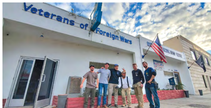
Local 40 RENEW Committee members helped with a complete rewiring and new light install at the Veterans of Foreign Wars in Burbank, CA.
